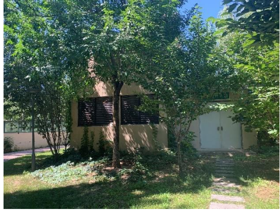
155 地块排风竖井 (2)
