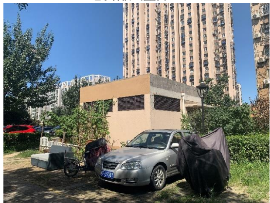
167 地块排风竖井 (6)
