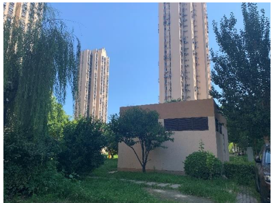
167 地块排风竖井 (8)
