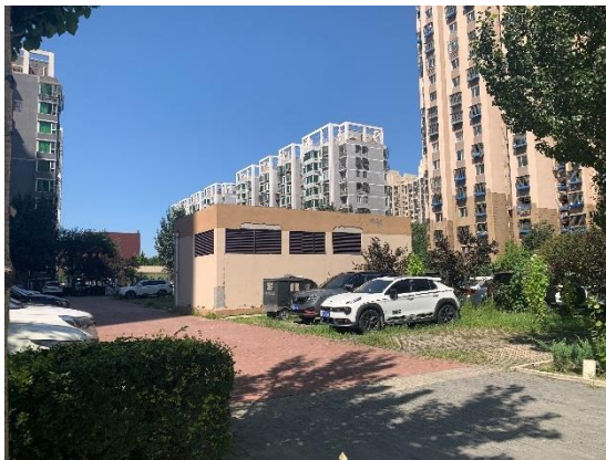
167 地块排风竖井 (7)
